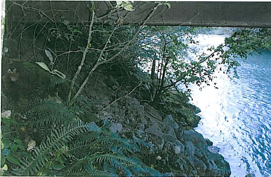
CK-2219 Left abutment
