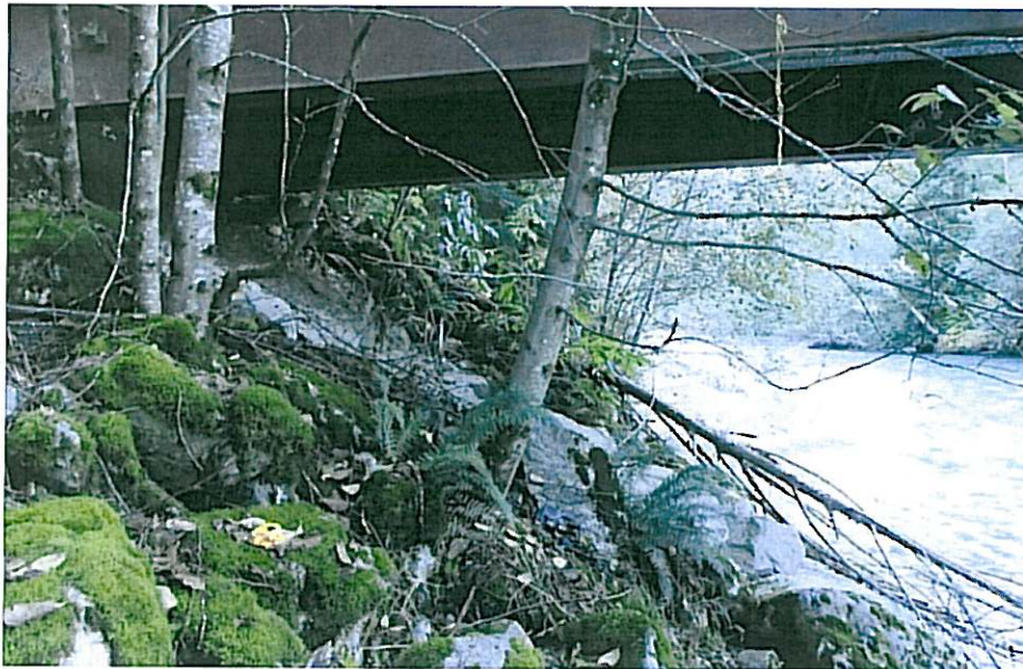
CK-2219 Right abutment
